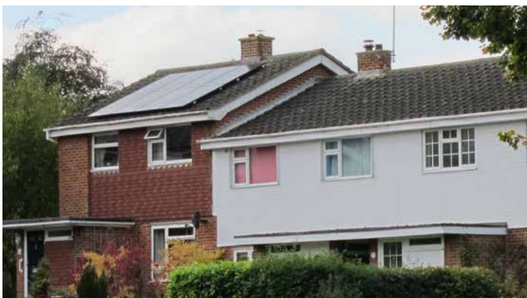
Local House with solar panels
